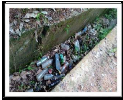
Improper Drainage System
